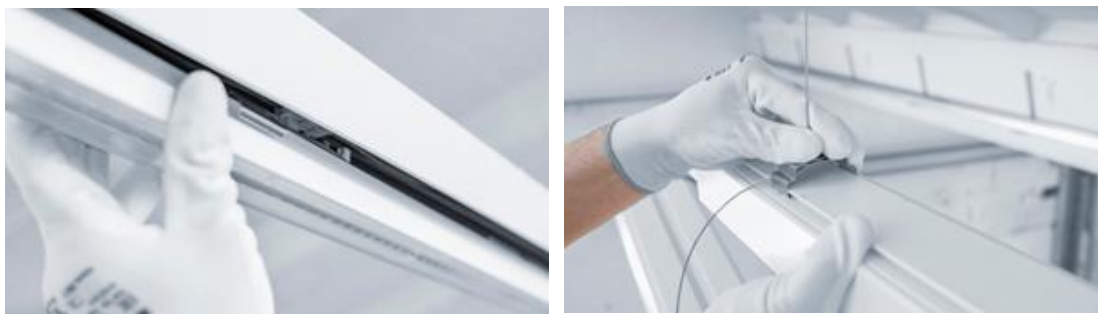
Fig. 3a + b: Up to 50 metres of the IP65 continuous-row system can be mounted in one piece. The trunking profiles, batten luminaires and lighting modules are all manufactured in metric dimensions.
